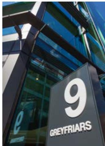
Reduced/minimal transoms assist limiting excessive material within façade design.
