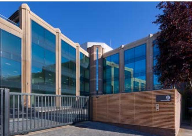
Deep plan window-to-window was designed to provide high levels of daylight throughout the floor plate. A high-spec glass was chosen in order to mitigate high solar gains on East to West elevations.
