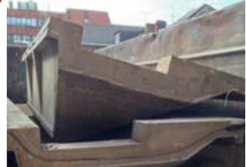
To successfully remove the cladding, the team went back to the original installers to determine how to remove the sections as a complete piece. Once we had established this they were able to remove them, eliminating the need to undertake crushing/breaking demolition. With this method of dismantling, the structure and floor plates were protected from damage.
